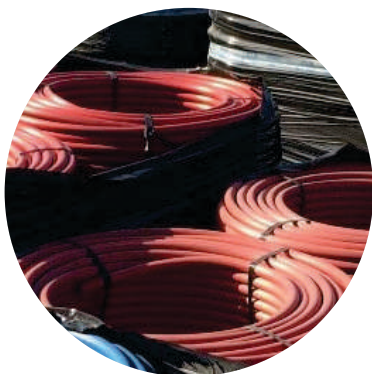
Channeling power cables in the building
